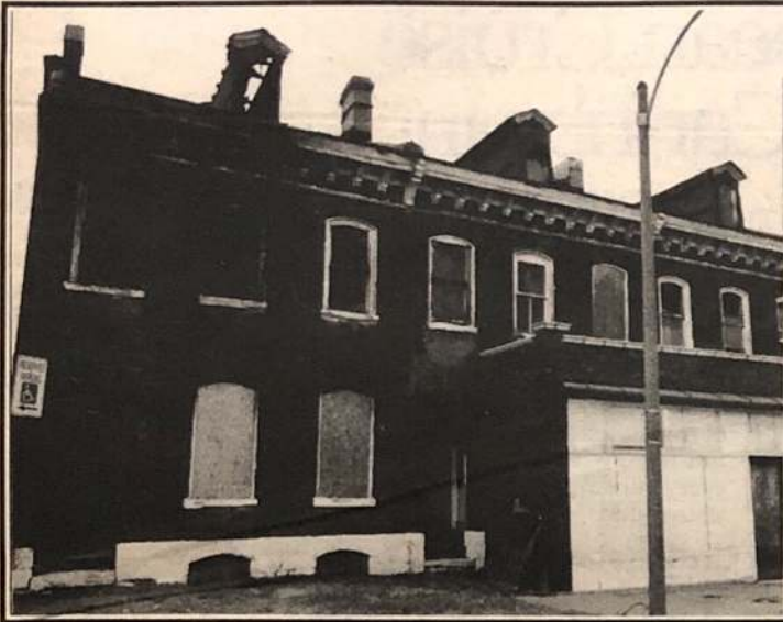
These three shells were hardly an inviting sight. In the throes of gut rehab, the storefront was removed, new floors, roofs and dormers were built. The historic cornice, windows and door were salvaged or recreated.
