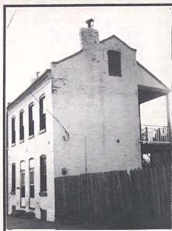
New homes will be modeled after this existing 19th century structure.
