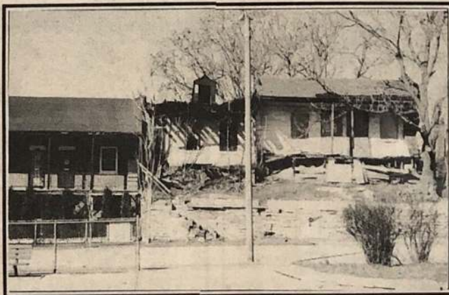
These dilapidated French Creole Cottages at 2211-15 So. Tenth were physical artifacts of St. Louis' pioneer days.
