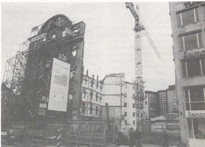
Gut rehab, German style: Everything but the facade walls is being rebuilt.
