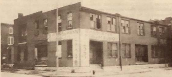
2357 S. 7th St.: 6 over 6 windows and massive doors define its industrial character.
