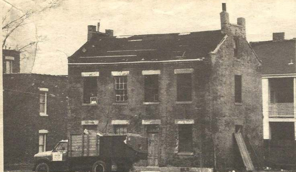
Front facade before rehab.
