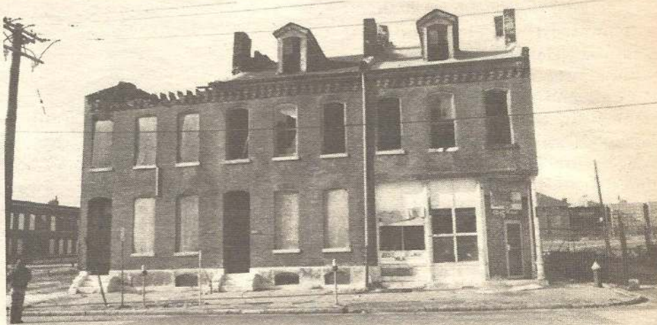
By the late 1970s, these buildings—and the Soulard neighborhood—were desolate and badly deteriorated. One rowhouse lost its roof!
