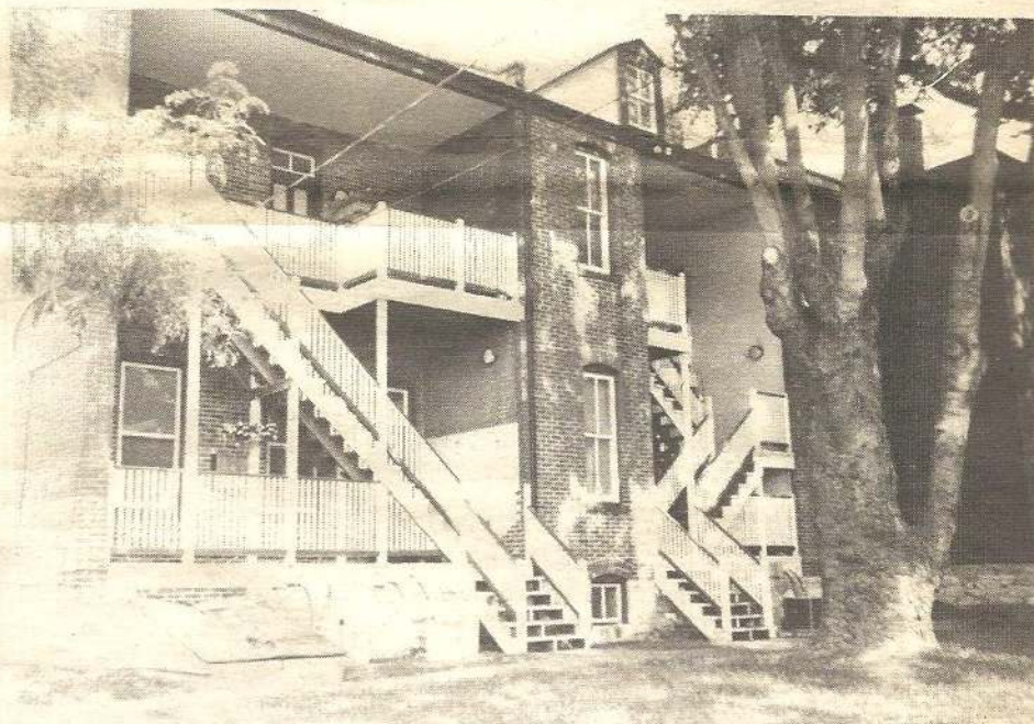
The rear porches of these multi-family rowhouses make their own interesting architecture.
