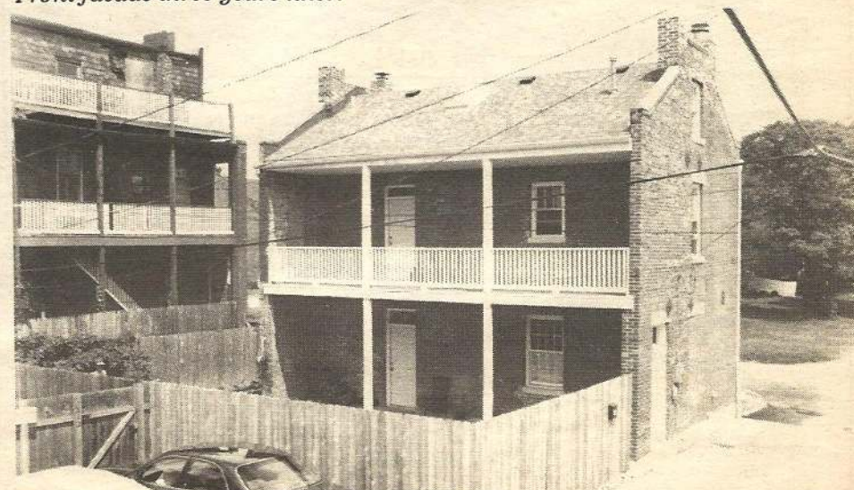
Restored porch and a fence around the yard!
