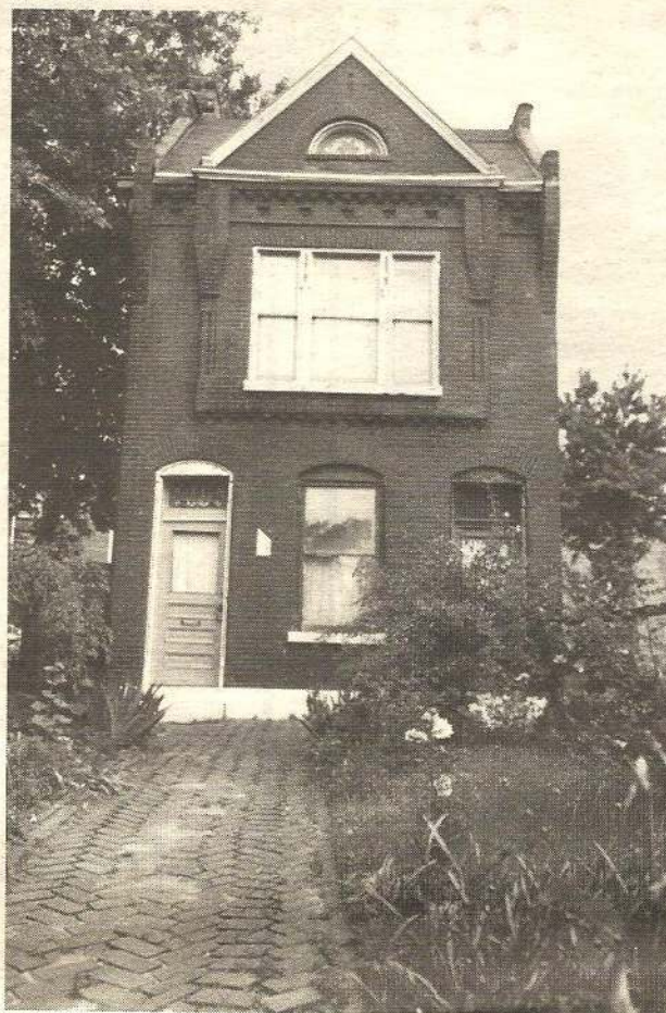
This home, shown as a shell on previous year's tours, has come a long way.
