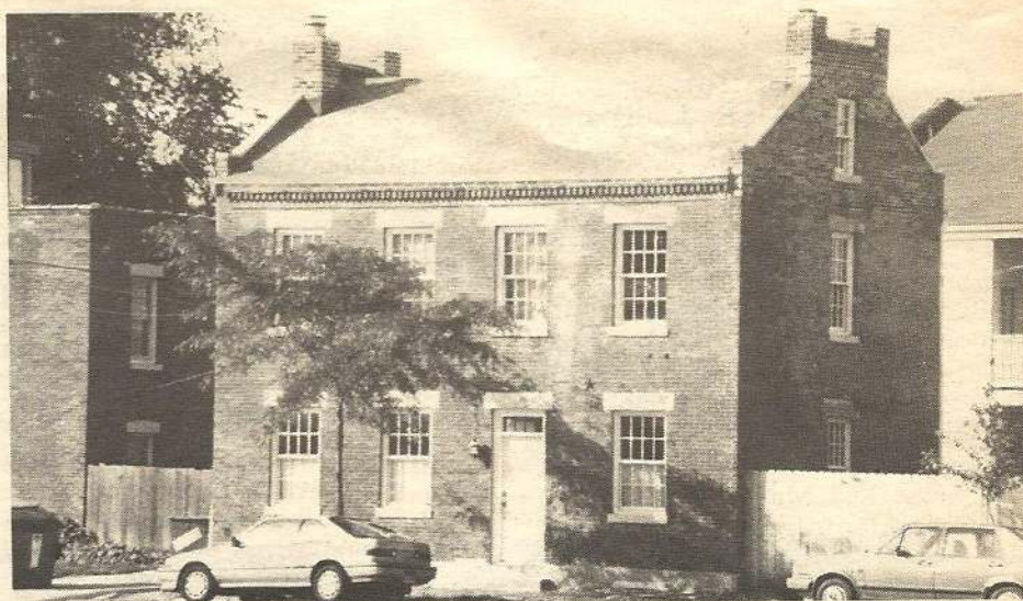
Front facade three years later.
