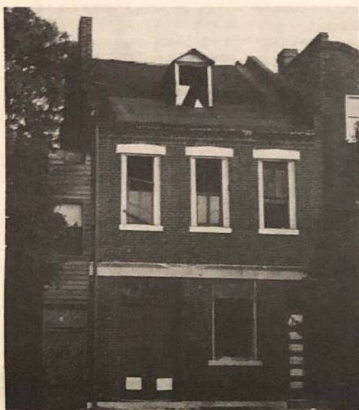
1834 S. 9th in 1988, before rehab.
