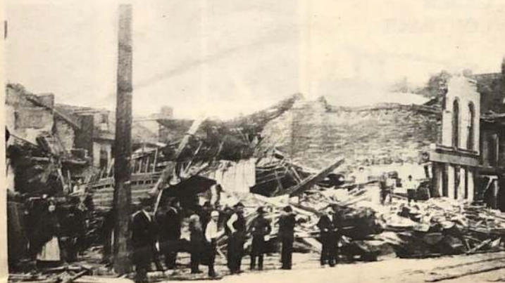
Broadway at Souland Street. Souland Market, one block west of this scene, was similarly wrecked.
