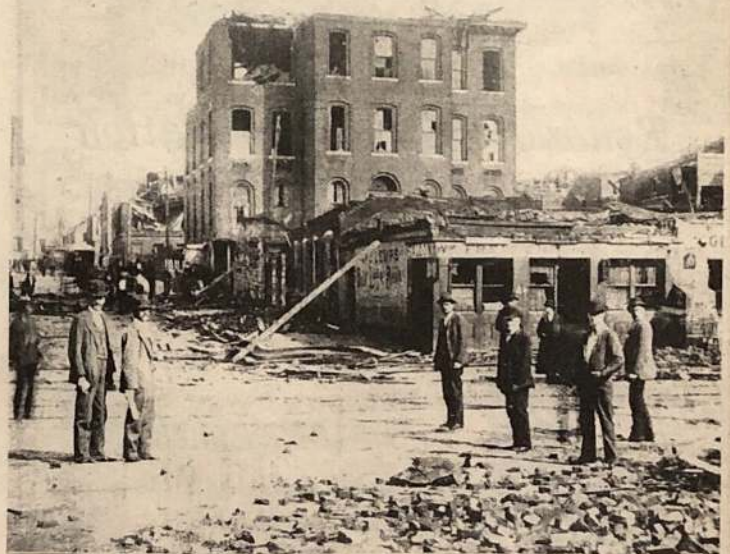
Corner of Broadway and Barry Street looking west. St. Vincent's Church in left background survived relatively intact.
