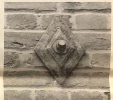
Diamond shaped cast iron brace.
