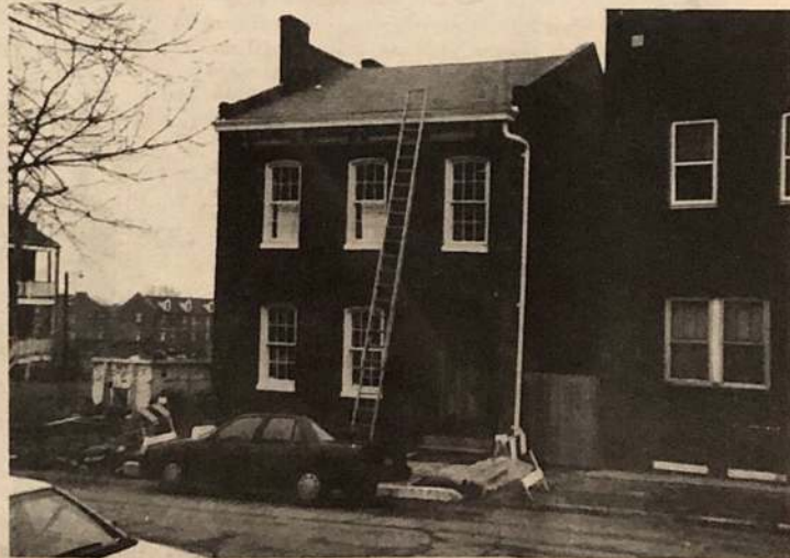
The finishing touches being added to this new/old home.
