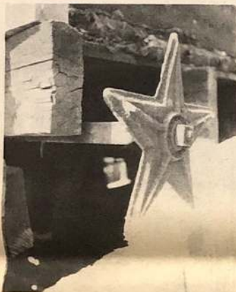
This wall under reconstruction shows a familiar 5-point star and the strap which connects it to the roof joist at left.
