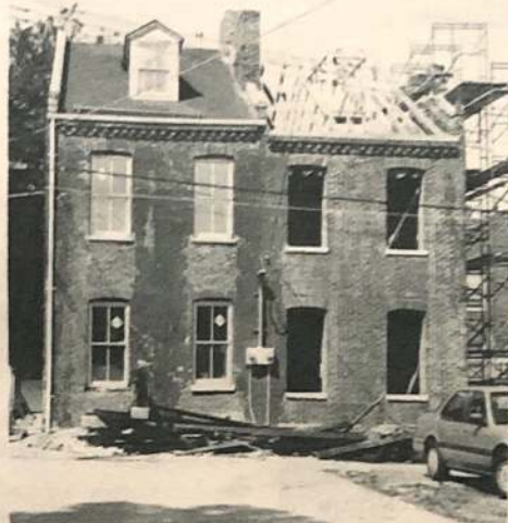
The same pair with rehab work well underway. 910 Rear Russell needed a brand new roof system.
