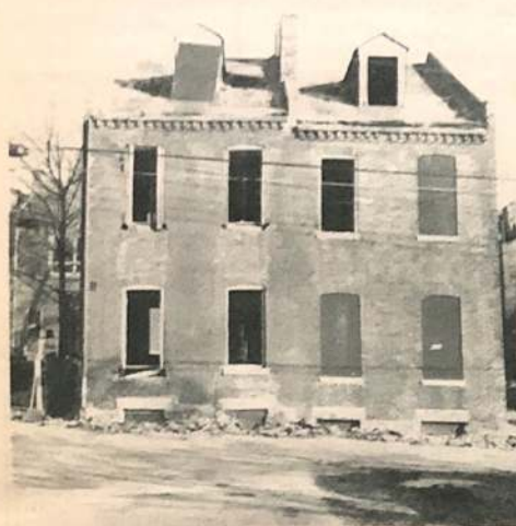
The alleyhouses at 910 Rear and 912 Rear Russell Blvd., as work was beginning.
