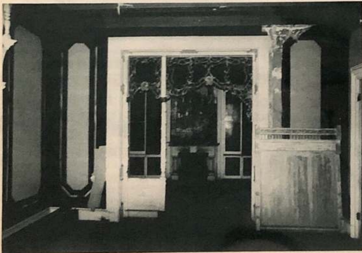
Gilded fretwork and canvas-covered walls (unfortunately painted over) in the parlor.
