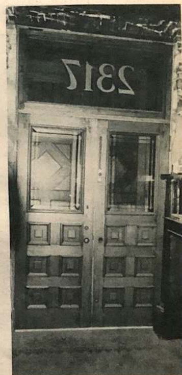
Massive oak double front doors, protected by another set of oak storm doors. All the glass is intact!
