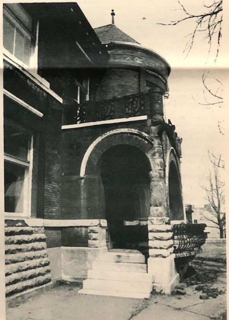
The heavy Romanesque porch dates from 1892, as does the turret. Note the different styles of foundation: The smooth foundation dates from 1875; the "rough" sections were overlaid in 1892.
