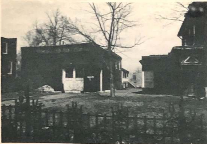
On the 1892 carriage house in the left foreground, one can still faintly see the painted sign "Carl I. Schaeffer Electric Co." The 1875 carriage house, with the porch, is in the background.
