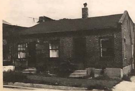
Dilapidated and unwanted, 1015 Geyer Avenue was seized for back taxes by the City.
