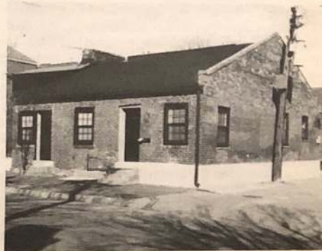
1015 Geyer Avenue Shines again as a finished two-bedroom cottage home.
