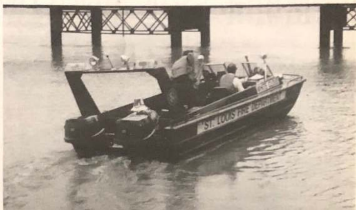
The White Cloud driving down Leonore K. Sullivan Blvd. during last summer's flood. —Photo courtesy of the Saint Louis Fire Department
