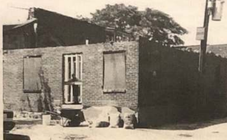
During rehab by Dave and Marge, the roof, all of the interior, and the back wall were razed. Then a new home was built within the remaining old structure.
