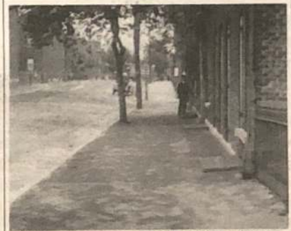
1920s street scene, exact location unknown. Note the herringbone brick sidewalk, the dirt/gravel unpaved street, and the limestone cobble gutter.
