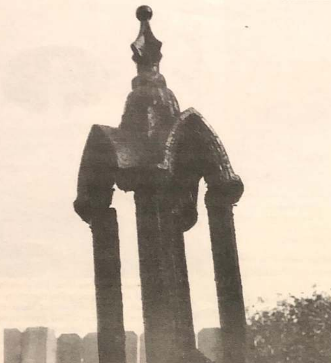
Fencepost, 12th Street at Shenandoah Avenue
