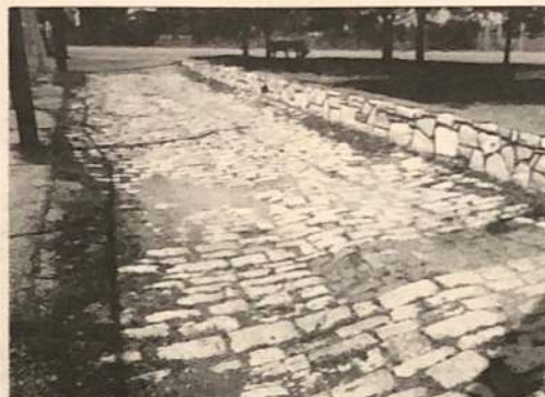
Here's the last exposed limestone cobble alley in the neighborhood. Go to the 2000 block of South 13th Street; this short stretch runs from 13th to Gravois, adjacent to a small greenspace park. This is what many European streets still look like.
