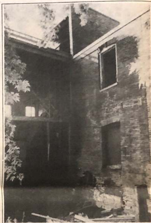
Crumbling wall just minutes before the main event.
