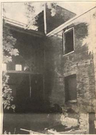
Crumbling wall just minutes before the main event.
