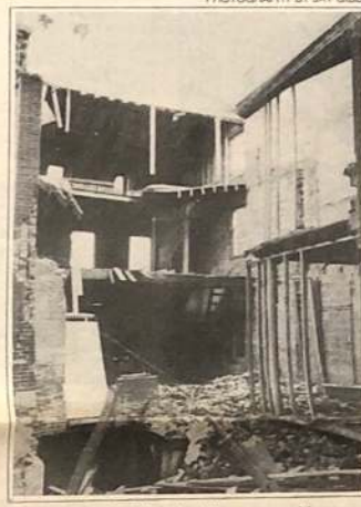
Same view, after floors had been removed by crane.
