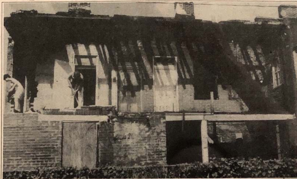
The original flounder house configuration emerges as Lori and friend dismantle a later addition.
