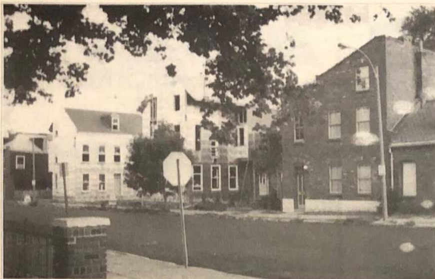
Infill houses under construction on the 800 block of Ann Avenue in 1984. Their next-door-neighbor is an old flounder house, an authentic Souard style.
