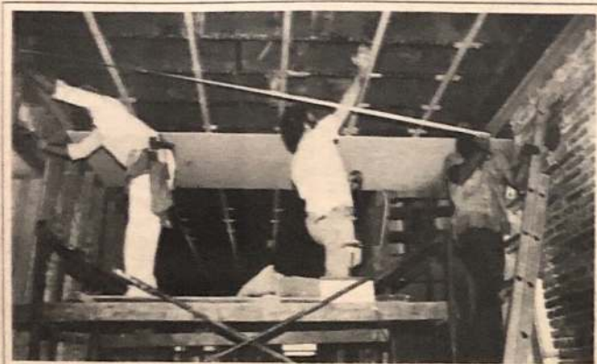
Contractor Bob, center, and helpers installing the first-floor ceilings. What a visual difference that was!
