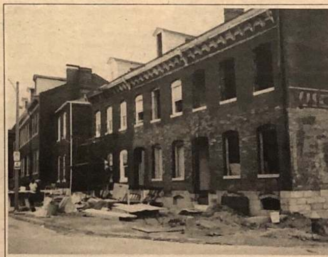
The restored 1880s façade. The replacement brick does not blend with the original—a problem still to be solved.
